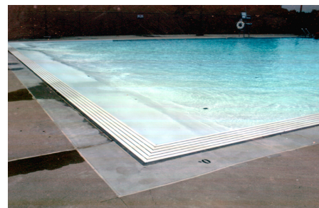
Rollout zero depth entry perimeter gutter system
